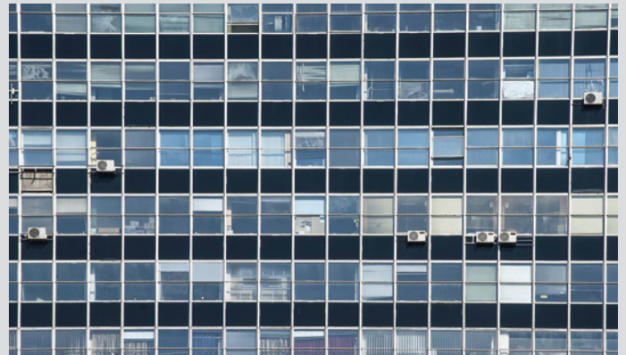
Reality – Internal blinds, lights on and localised AC units
